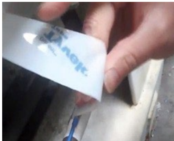
Figure 46. Wrap RTD sensor with Tyvek tape
