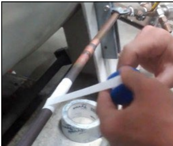
Figure 44. Wrap Teflon tape around 3" Section of LN 2 fill line
